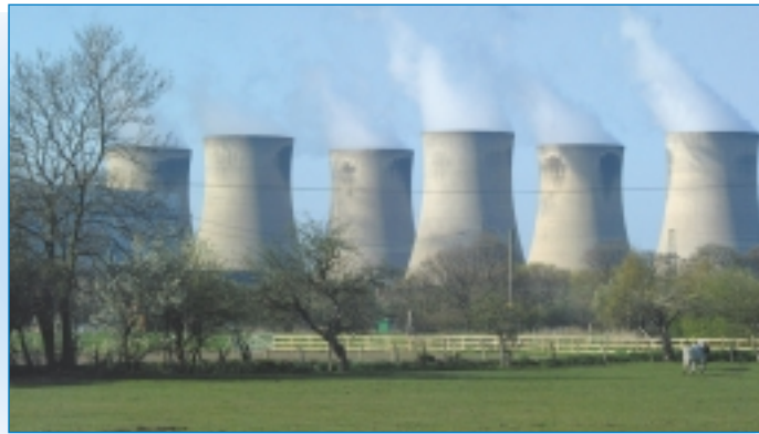
Drax is the largest coal-fired plant in Western Europe, and produces more than eight percent of all electricity generated in England and Wales.
